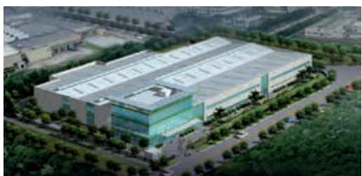
Schneider Busway (Guangzhou) Ltd. is certified having ISO 9001 quality management system, ISO 14001 environment management system and OHSAS 18001 occupational health and safety management system.
